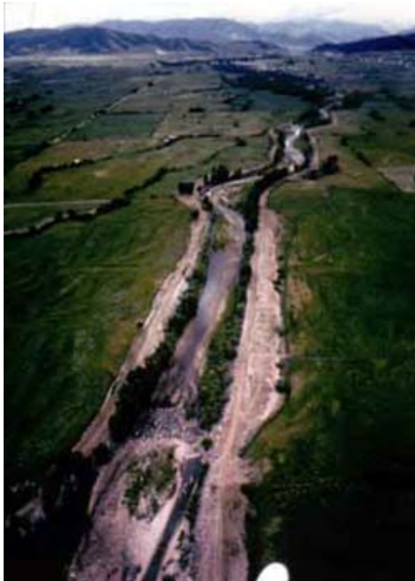
Figure 13 The pre-Jordanelle channelization of the river. From Provo River Restoration Project .
