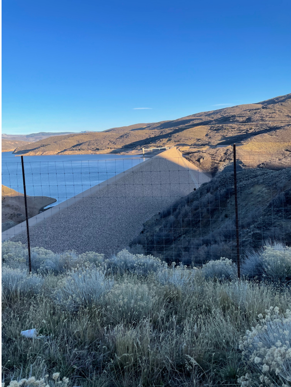
Figure 4 Photo of the Jordanelle dam looking east. In the far distance is the SLOW tower that feeds the dam penstock through one or more of the tower's inlet gates located at different levels in the water.
